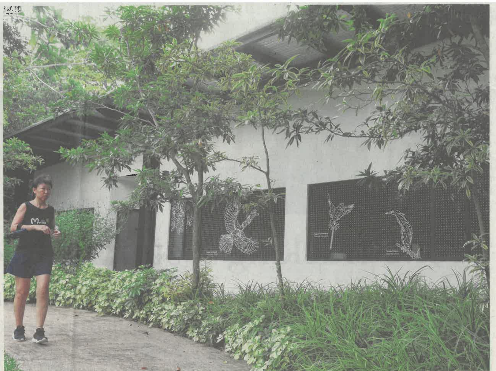
Frosted glass film and decals applied to the windows of the Hands-On House at HortPark. This minimises reflection and reduces light transmission, which will, in turn, prevent birds from flying into the windows. A 2017 study found 237 migratory birds crashed into buildings here between 1998 and 2016. ST PHOTO: KELVIN CHNG
